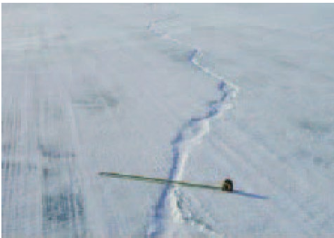
Longitudinal ice contraction crack
