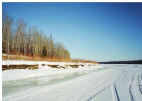
Evidence of wet cracks underneath a snowbank from water that flowed through the cracks and froze on the surface
