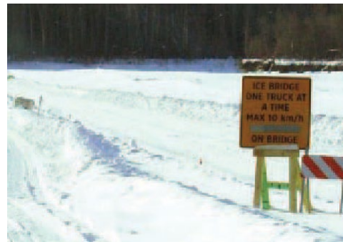
Sign that limits travel on the ice bridge to one vehicle at a time
