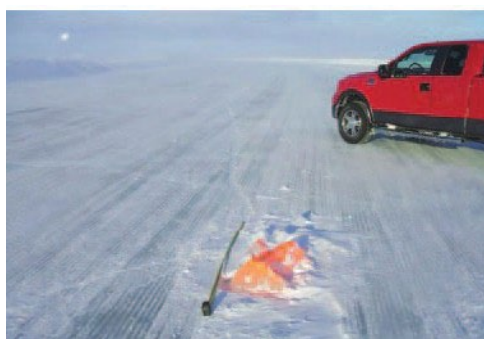
Longitudinal cracks that have intersected and caused a block of ice to pop out
