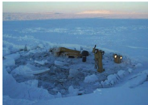
Breakthrough of a D10 Caterpillar tractor following formation of a circumferential crack pattern
