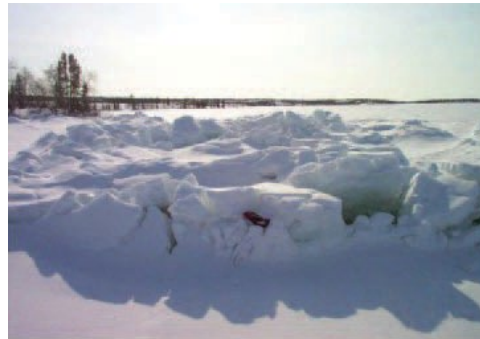
Blowout caused by speeding vehicles creating dynamic waves that release their energy at weak areas in the ice
