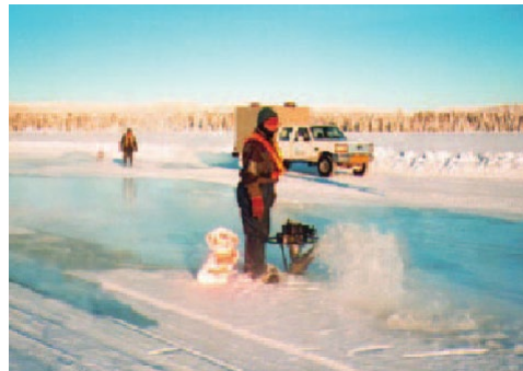
Flooding crew repairing an ice road
